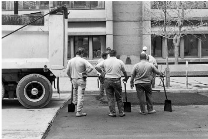
Construction watchers, Montréal, 1997
